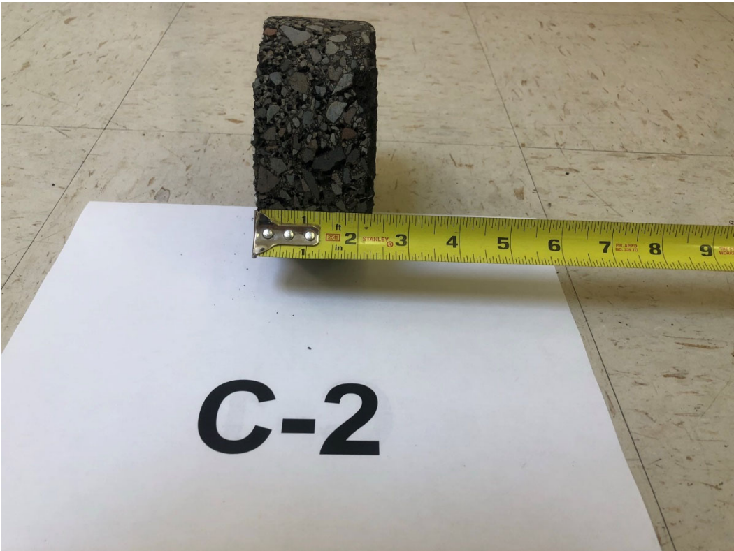
Photo 2. Pavement Core C-2
