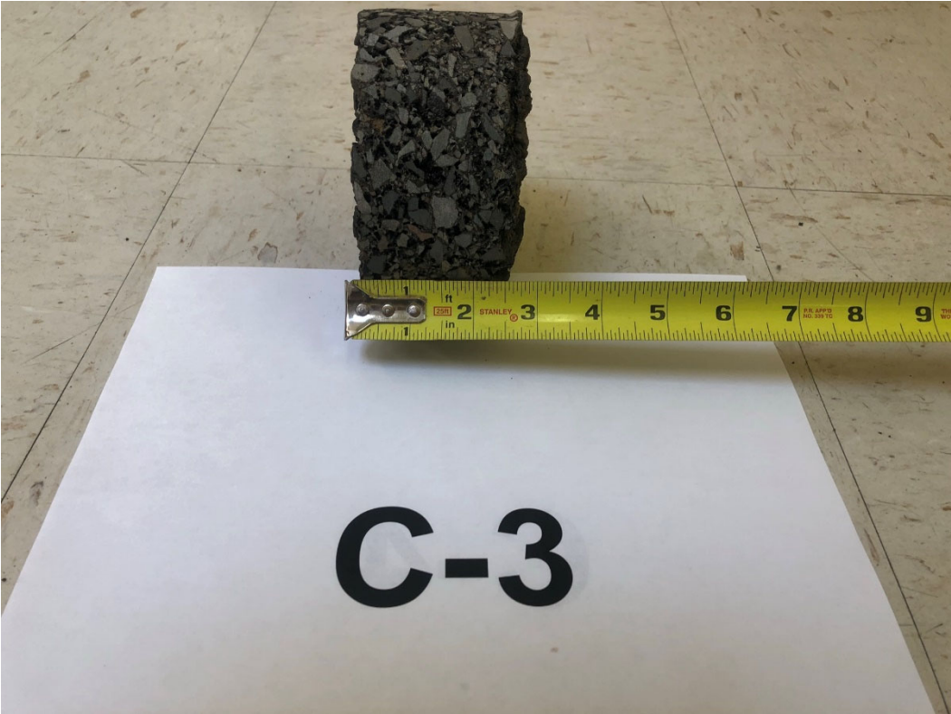
Photo 3. Pavement Core C-3
