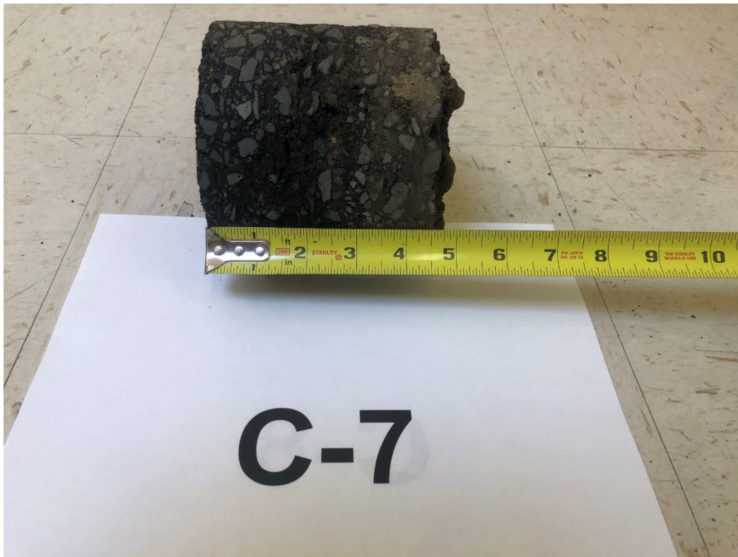
Photo 7. Pavement Core C-7
