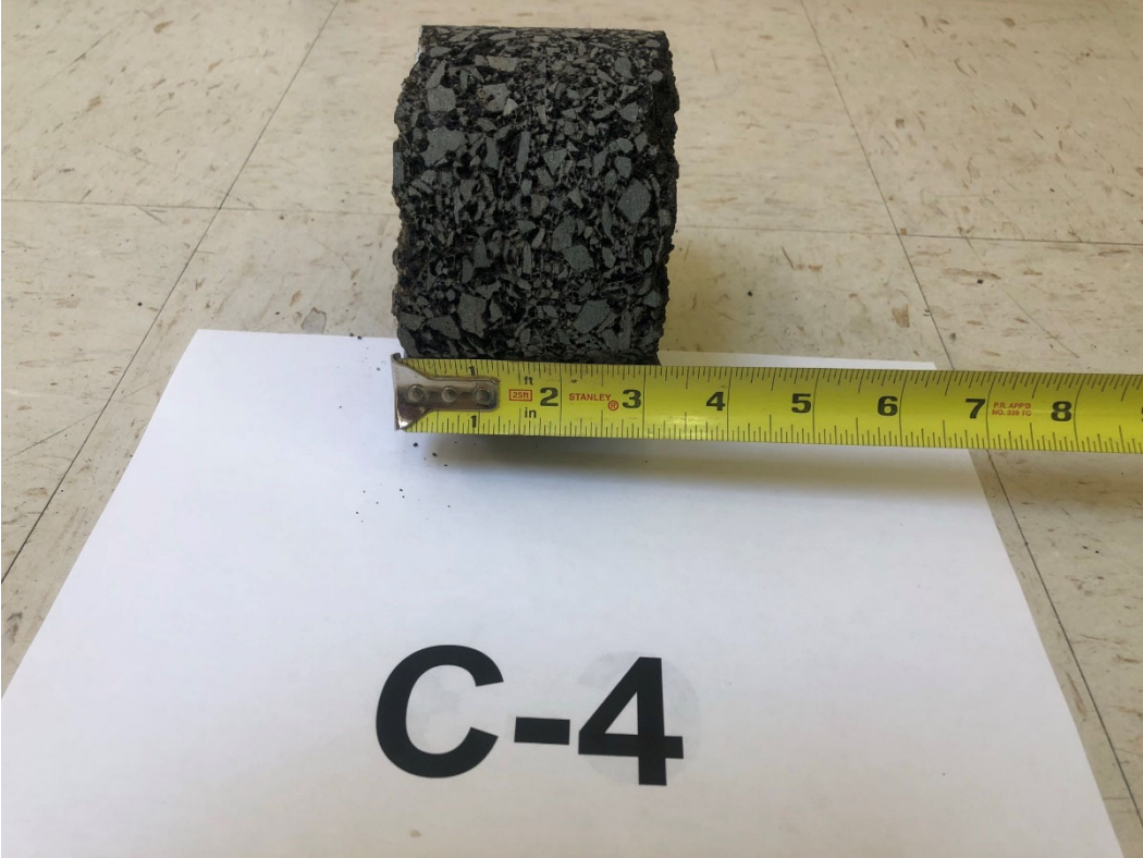
Photo 4. Pavement Core C-4
