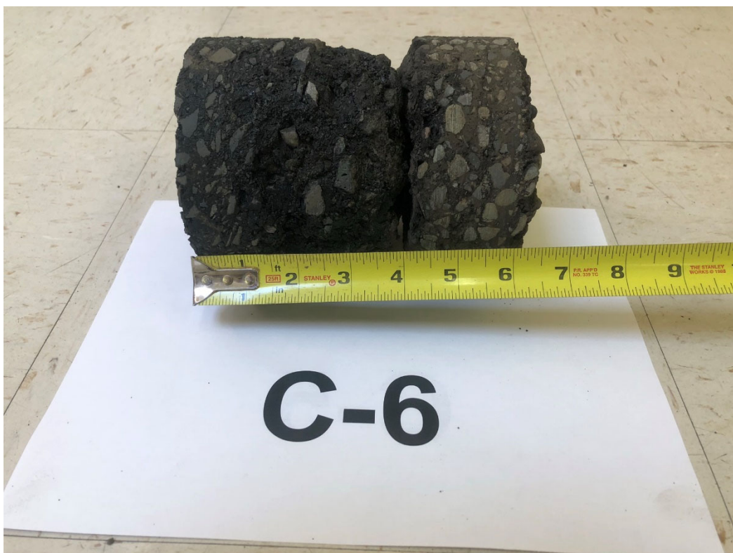
Photo 6. Pavement Core C-6
