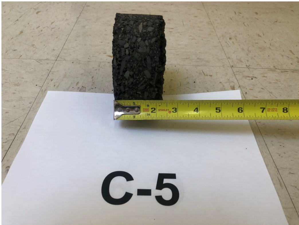
Photo 5. Pavement Core C-5 ( Note: 6" core thickness estimated based on drilling)
