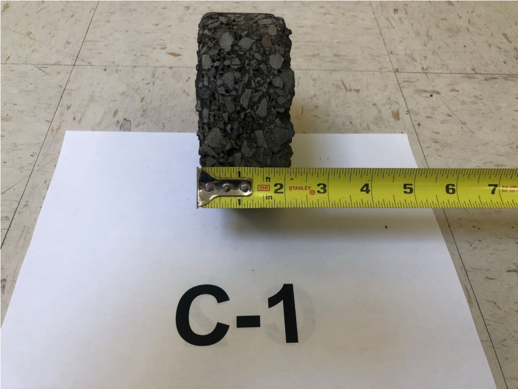
Photo 1. Pavement Core C-1
