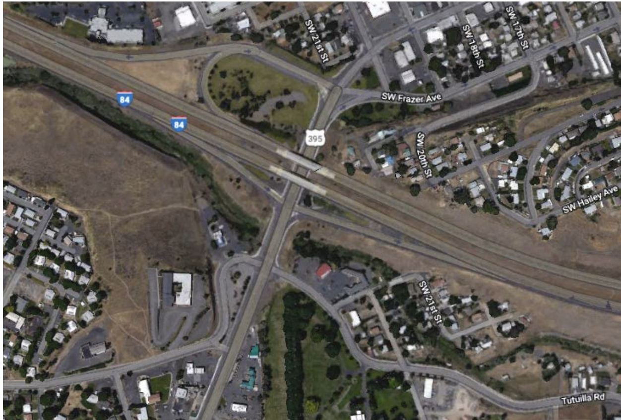
North and South Side of Current Southgate Interchange
