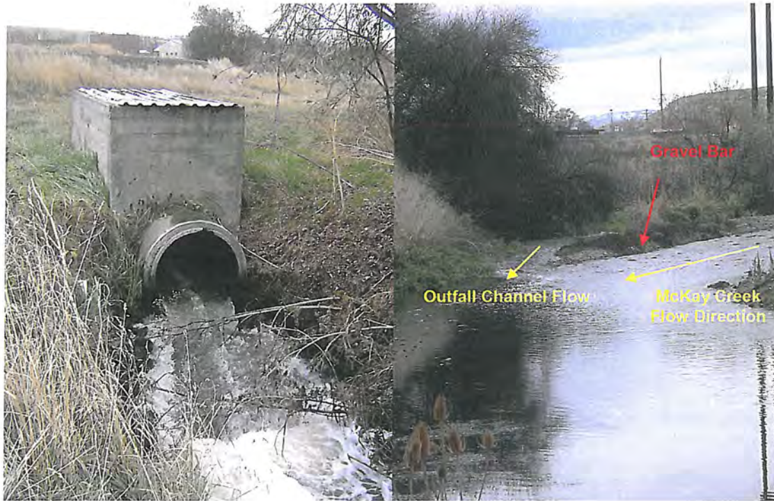
Figure 9. Existing Outfall Channel
