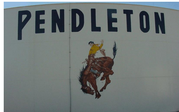
Water Treatment Plant Water Tank
