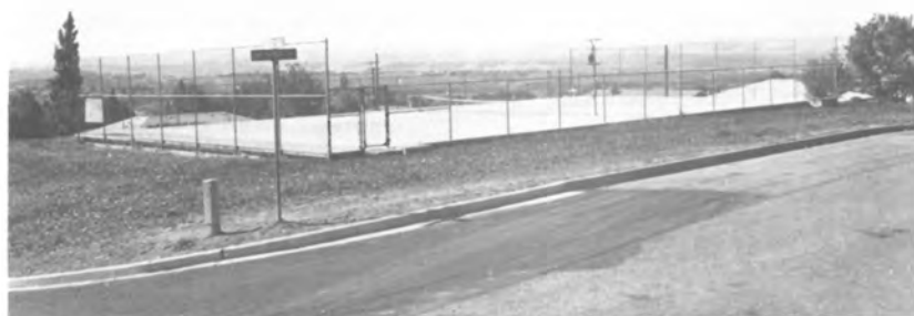
NORTH HILL RESERVOIR
