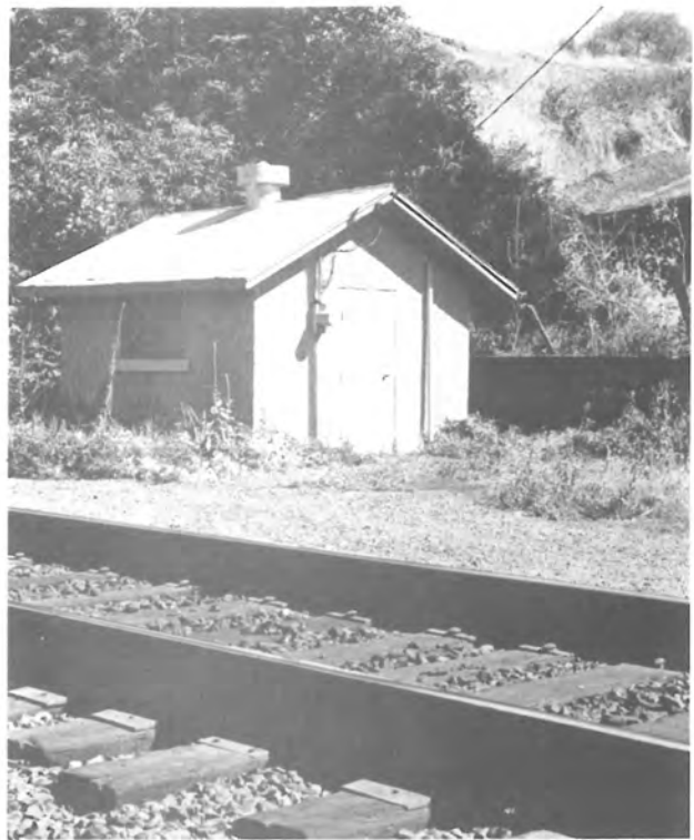
WEIR HOUSE BELOW WENIX SPRINGS
