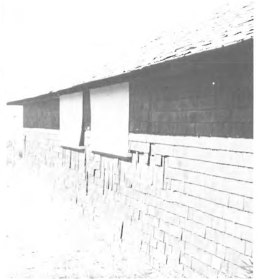
SOUTH SIDE EXTERIOR
