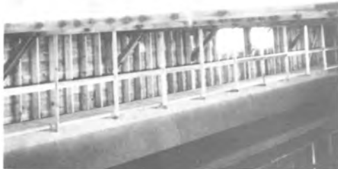
INTERIOR - WEST RESERVOIR SOUTH HILL RESERVOIR
