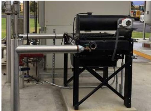
850 Cogeneration - Waste Heat Radiator
