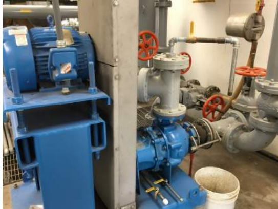
763 Secondary Digester Mixing Pump
