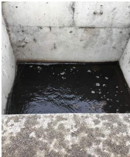
470 Effluent Junction Box
