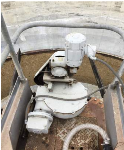
451 Secondary Clarifier East Drive
