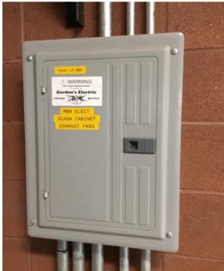
439 MBR Building Lighting Control Panel
