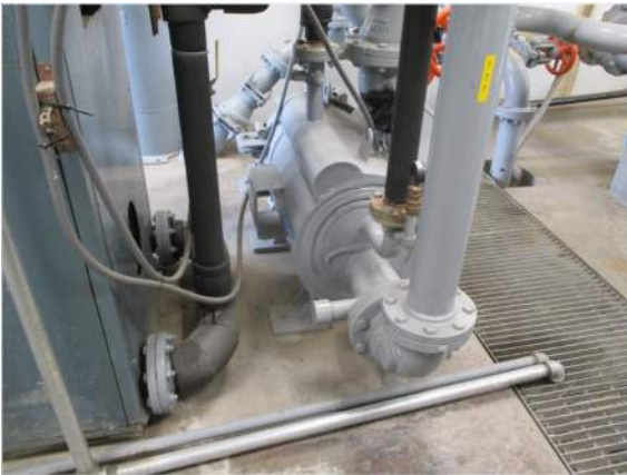
766 Secondary Digester Heat Exchanger
