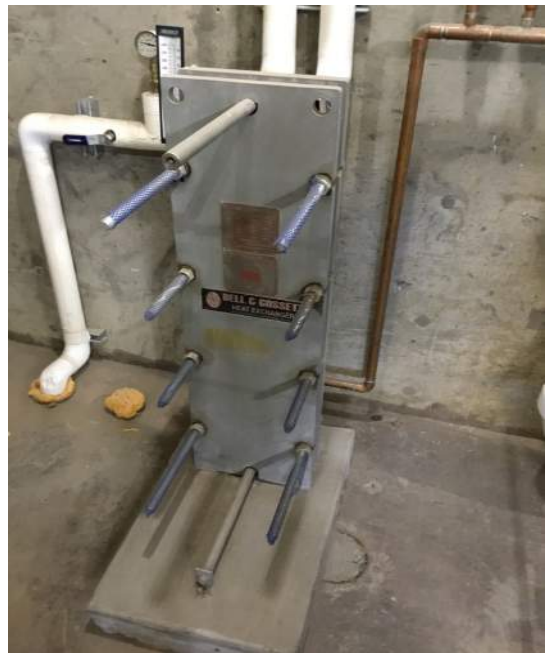
814 Washdown Heat Exchanger
