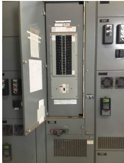
636 Dechlorination Building Lighting Power Panel
