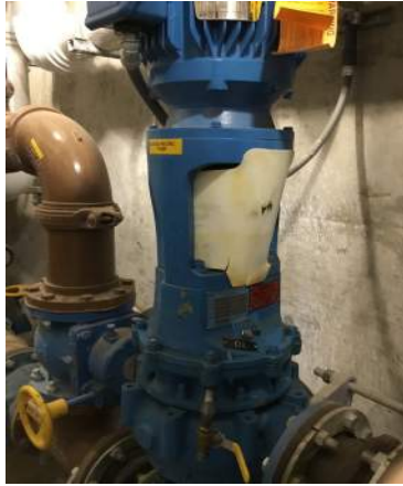
709 Primary Digester Sludge Recirculation Pump
