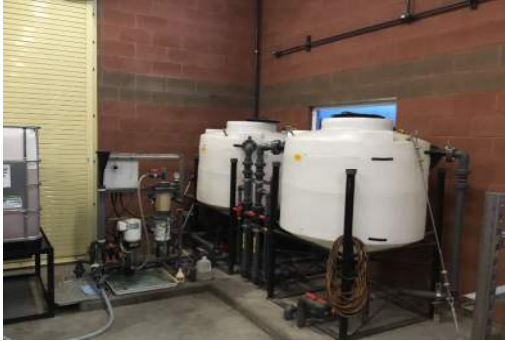
788 Dewatering Polymer System
