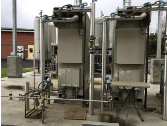
850 Cogeneration - Microturbines
