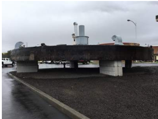
762 North Secondary Digester Floating Cover
