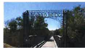
A new pedestrian and bicycle bridge at 4th could be included as part of this project to create a connection to the existing River Walk at Pioneer Park.
