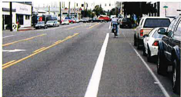
Typical bike lane on urban higher speed/volume roadway
