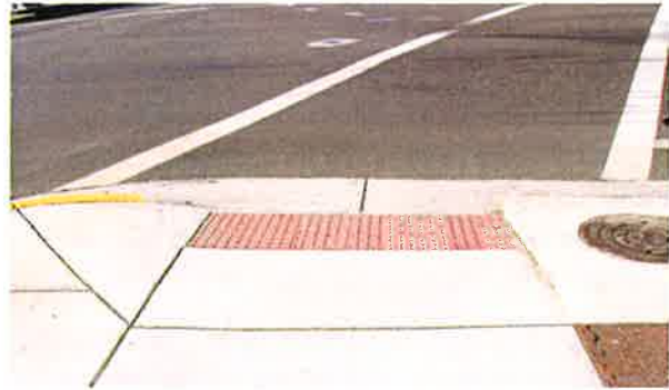
Curb ramp with one flare
