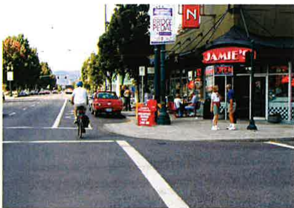
Removing a travel lane created room for a bike lane, curb extension and on street parking
