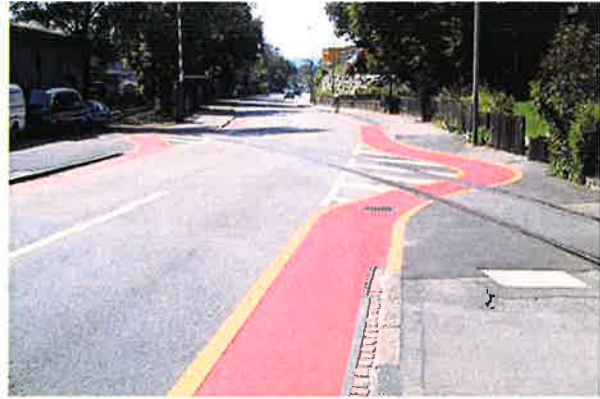
Rail crossing S curve
