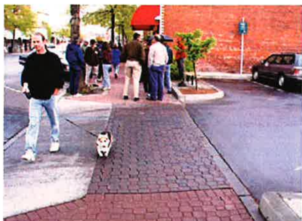
Sidewalk thru alley entrance is kept level
