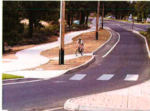
Bicyclist using exit ramp to access sidewalk
