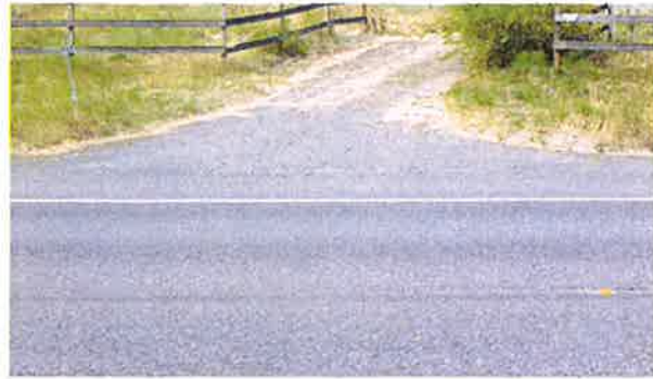
Paved driveway apron keeps gravel off shoulder
