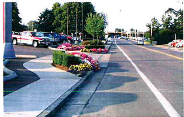
Sidewalk is kept level at driveway
