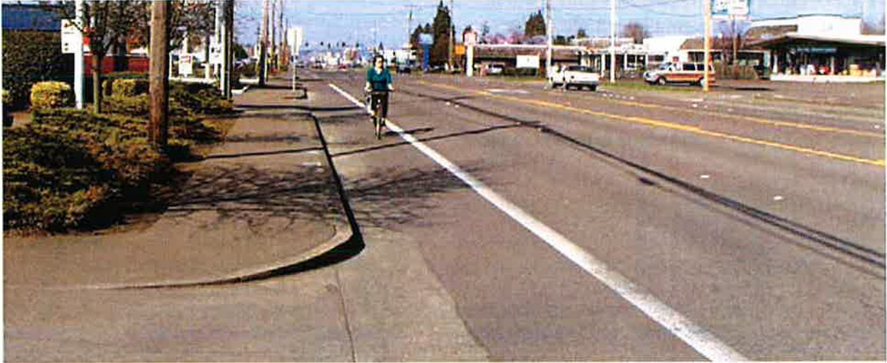
Bike lane restriped by narrowing travel lanes on commercial arterial
