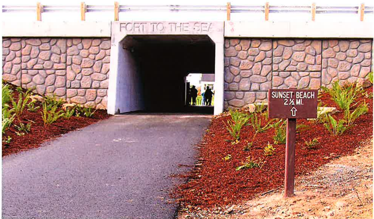
Undercrossing with good sight lines
