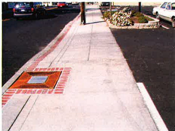
Dustpan style driveway approach improves pedestrian safety
