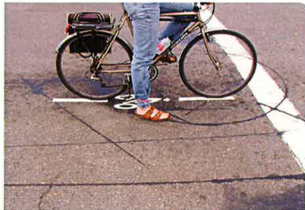
Stencil indicates where to position bicycle over loop detector to trip signal
