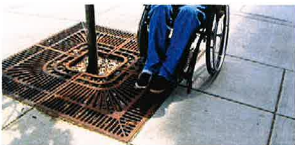
Wheelchair traversable tree grates may extend into pedestrian zone
