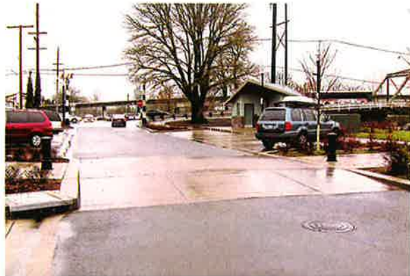
Raised intersection keeps crossing level with sidewalk
