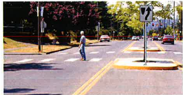
Median island provides mid-street refuge for pedestrians
