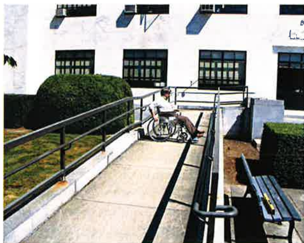
Level landing provides resting area
