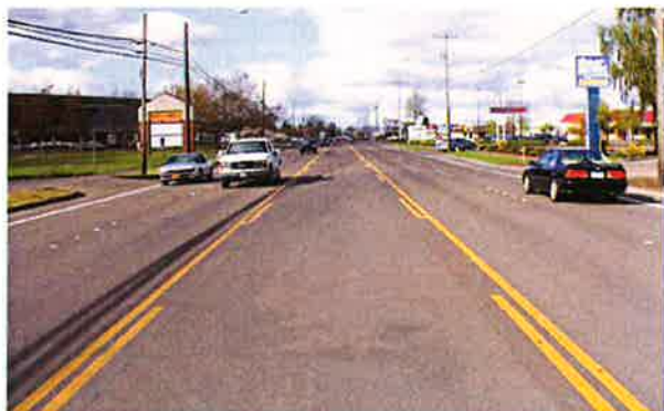
A wide, multi-lane street built for motor vehicle capacity is difficult to cross
