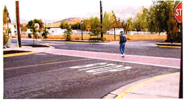
Textured crosswalk with supplemental white markings
