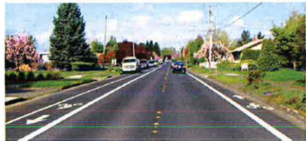
Parking removed from one side to add bike lane
