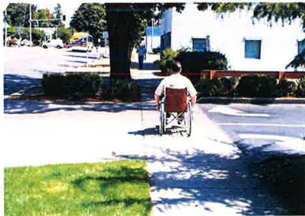
Separated sidewalk stays level at driveways and is free of obstacles
