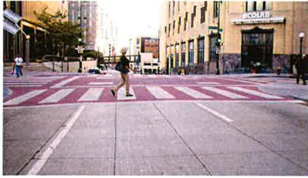
White markings inset into colored pavement
