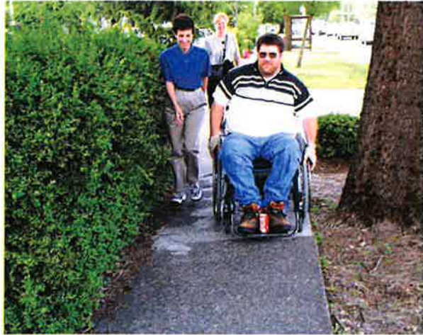
5 foot sidewalk is uncomfortably narrow
