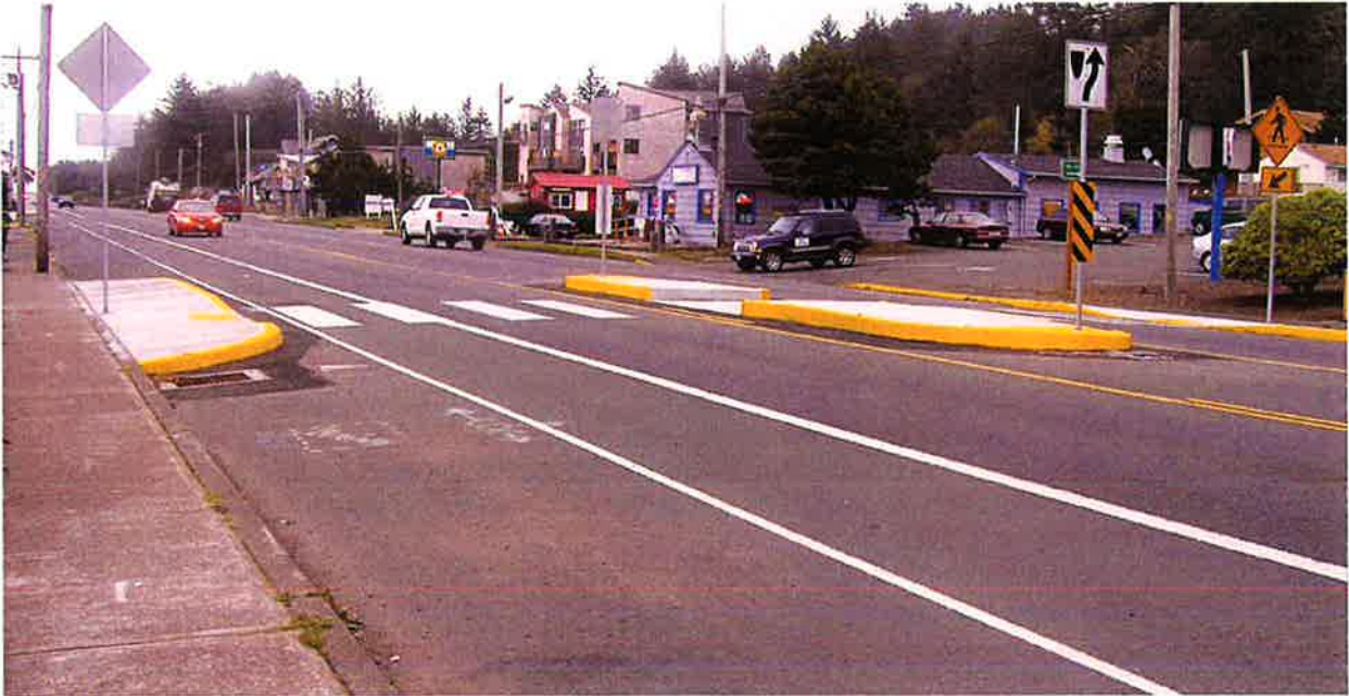
A successful pedestrian network requires safe and convenient crossing opportunities
