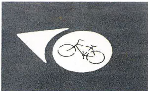
1st Generation bicycle boulevard pavement marking
