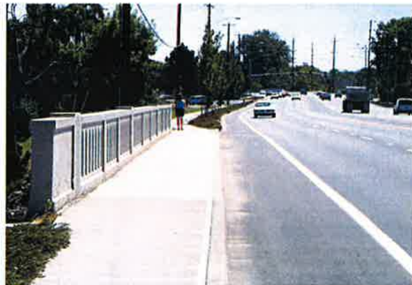
Furniture zone eliminated at pinch point
