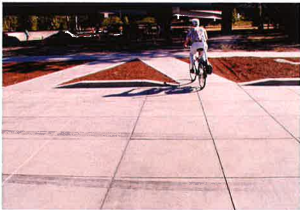
Split path entry eliminates need for bollards
