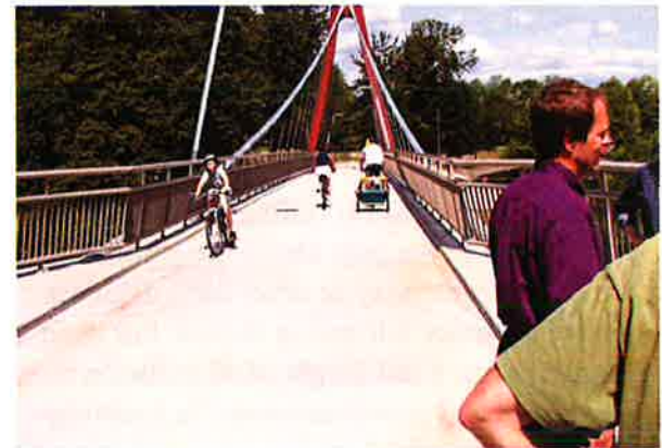
Pedestrians stop to admire the view in widened area without impeding thru traffic
