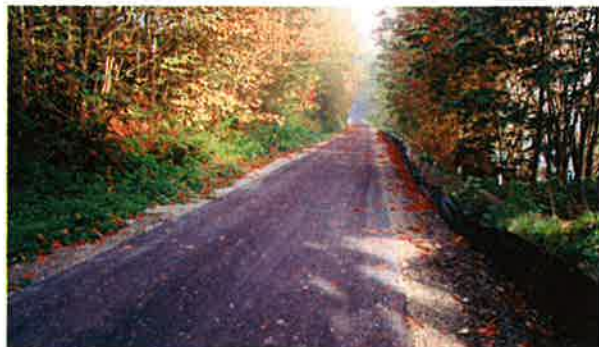
Gravel shoulders prevent raveling of path edges
