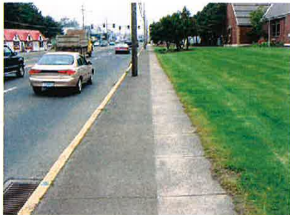
Sidewalk widened to 6 feet
