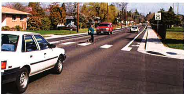
Painted crosswalk on two lane roadway is appropriate
