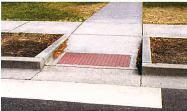
Perpendicular Curb Ramp
