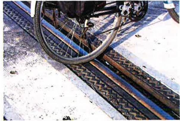
Concrete RR crossing with rubber flanges
