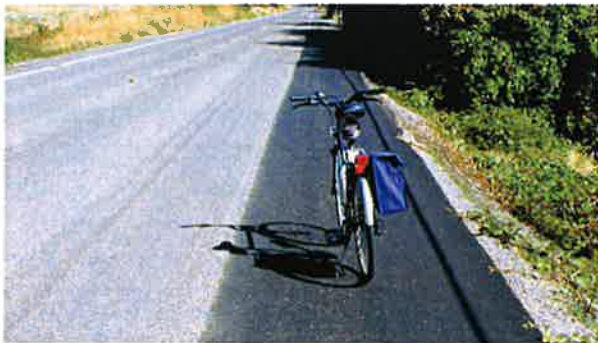
Chip seal ends at motor vehicle travel lane
