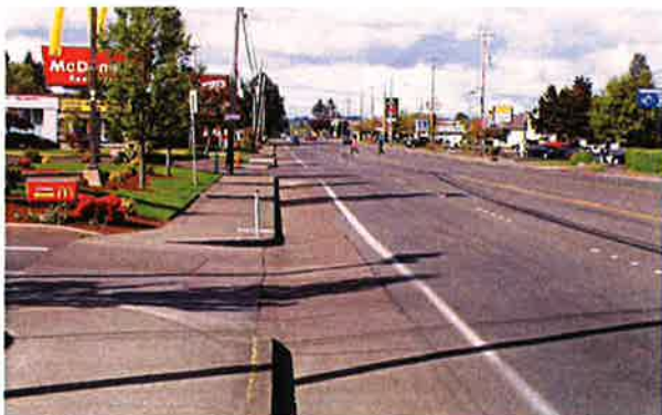
It is difficult to determine where pedestrians will cross on auto oriented streets with diffuse destinations
