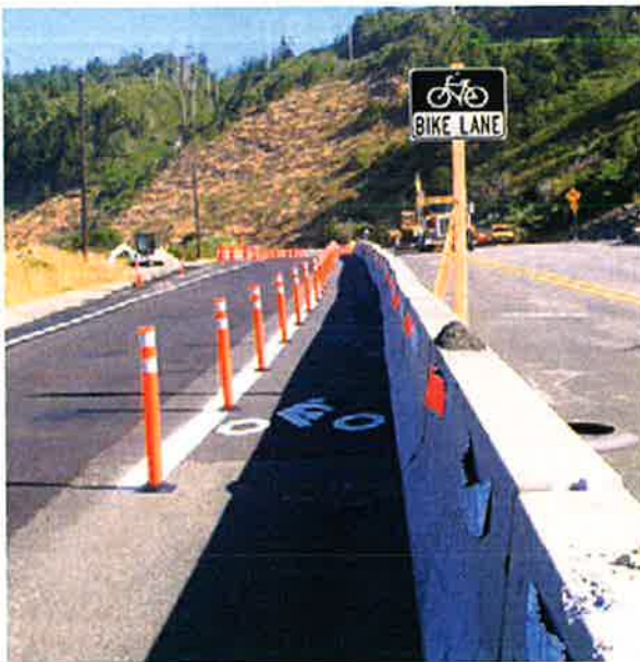
Bike lane in temporary work zone
