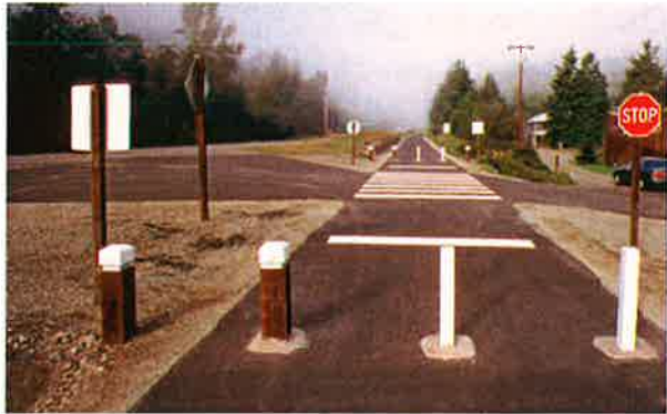
Path crossing a minor street should have been given priority right of way
