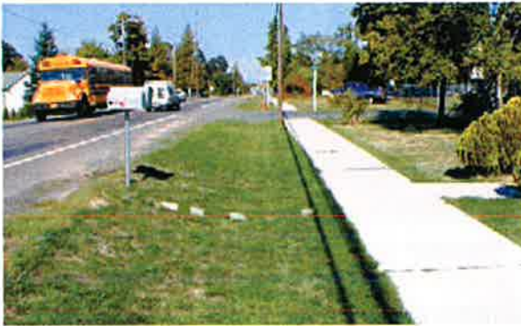
Sidewalk behind swale
