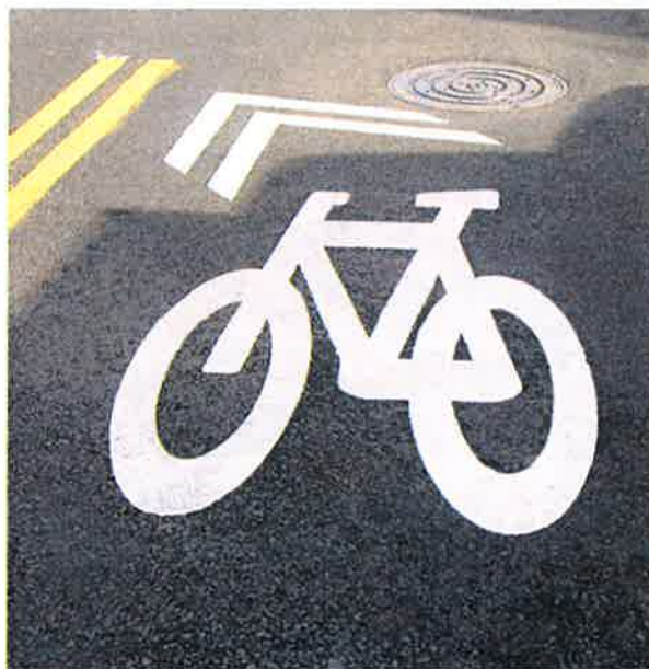
2nd Generation bicycle boulevard pavement marking (indicates turn)
