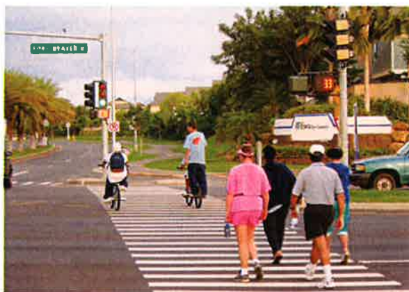
Pedestrian signal head in line with crosswalk
