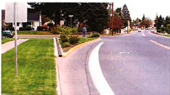
Formerly skewed intersection realigned to right-angle
