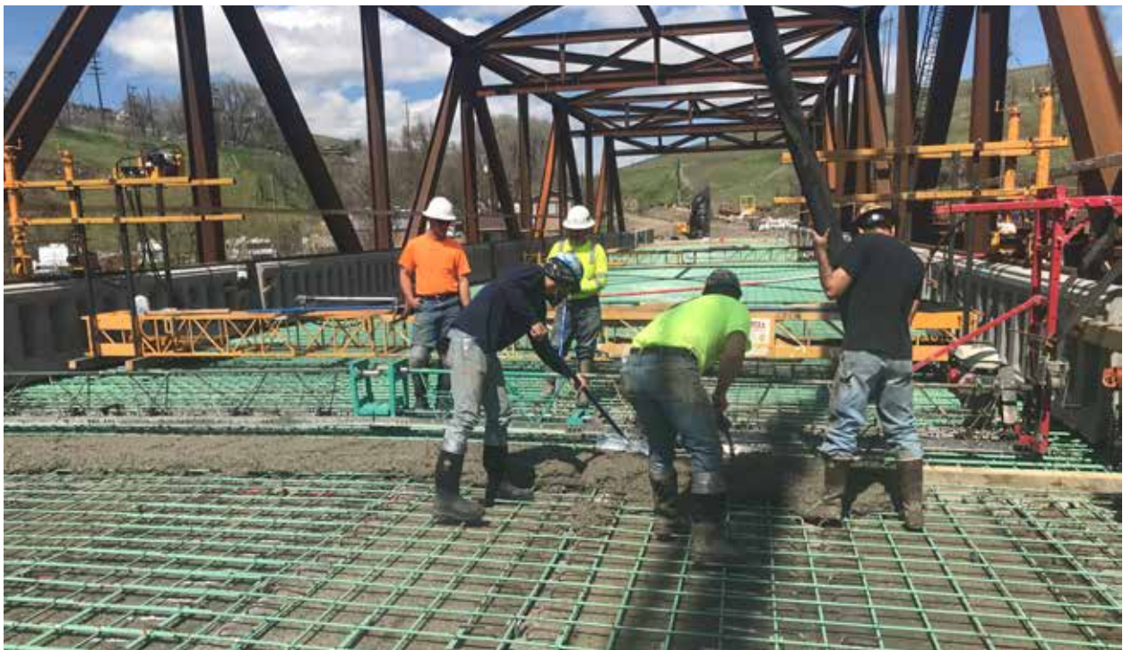
▼ Crews pouring the concrete deck
