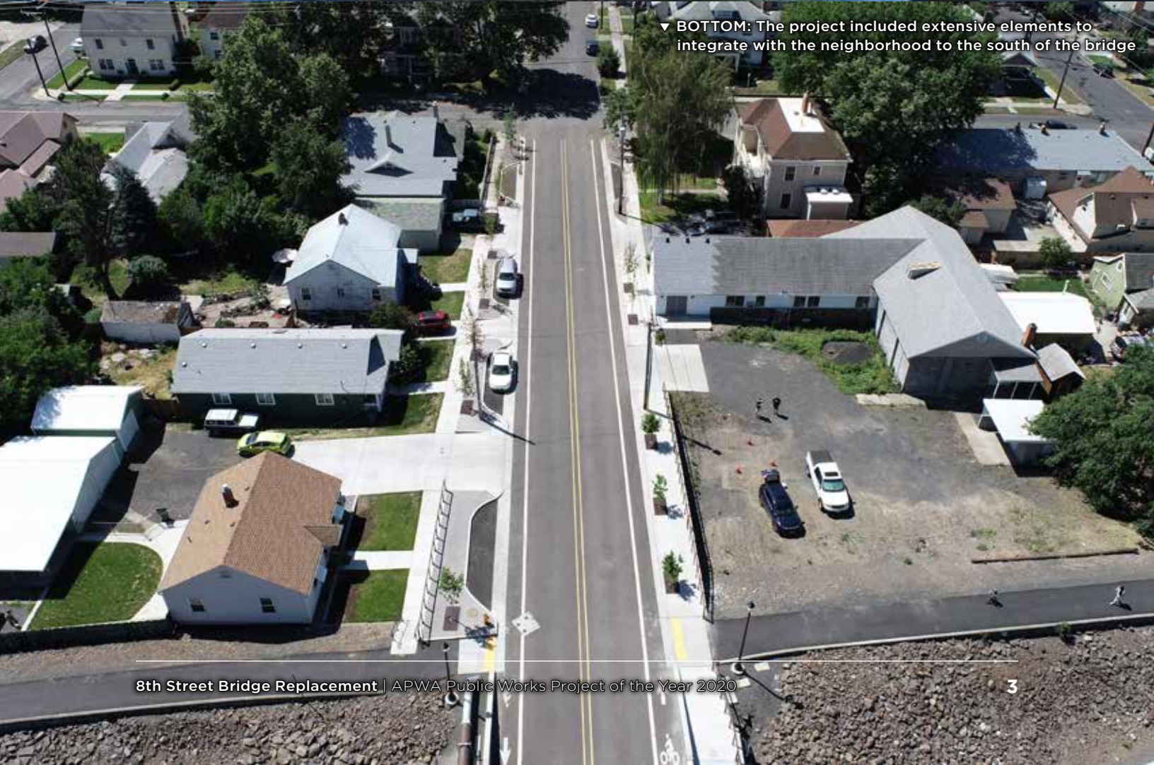
▲ TOP: Final constructed bridge as seen from the west.
