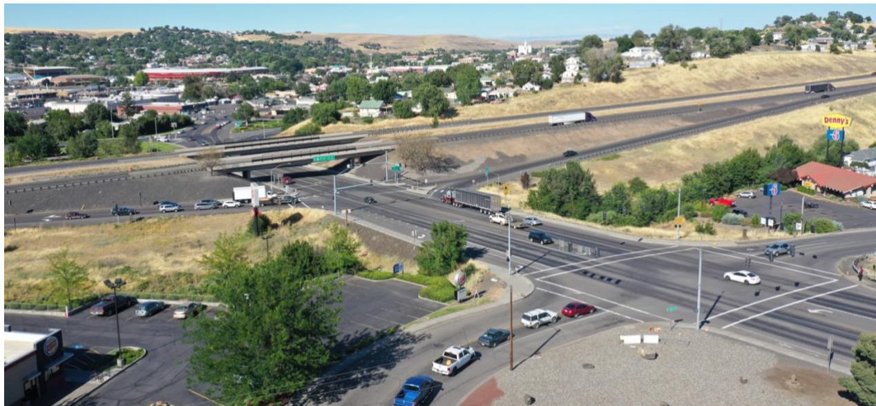
Southgate Interchange viewed from the south during non-peak hours
