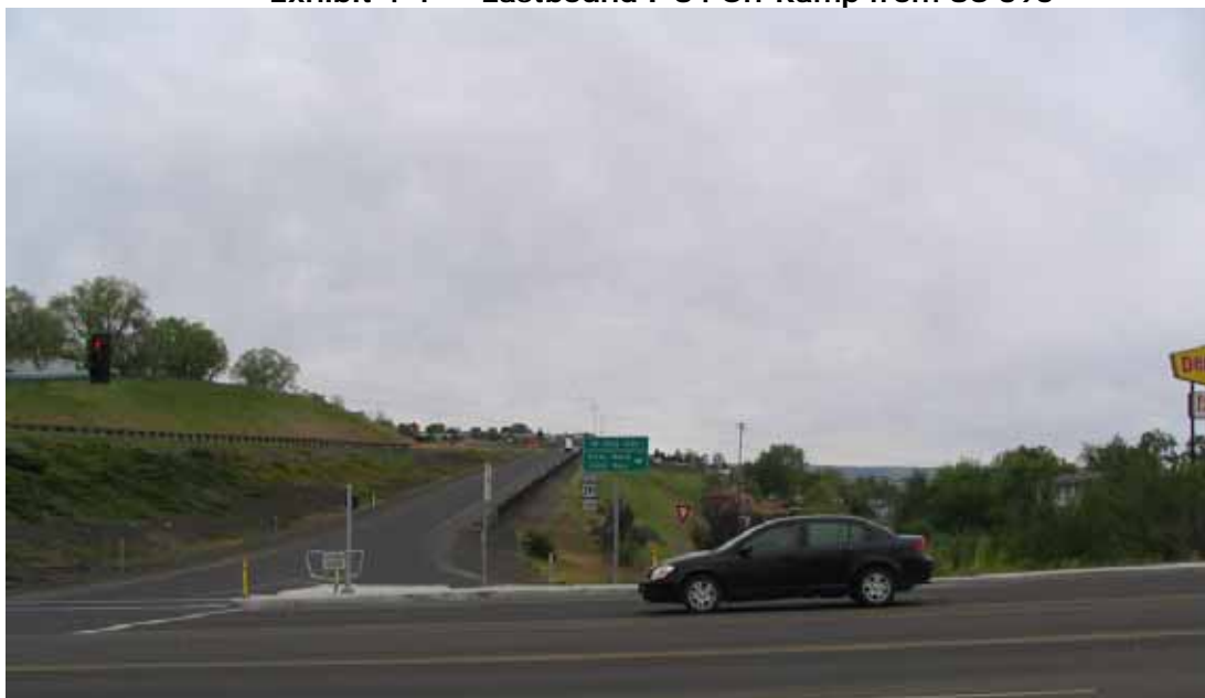
Exhibit 4-1 Eastbound I-84 On-Ramp from US 395
