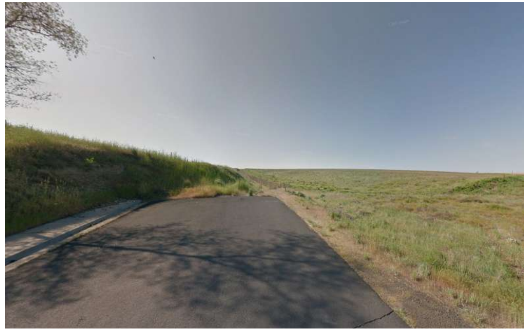
④ VIEW LOOKING SOUTH
