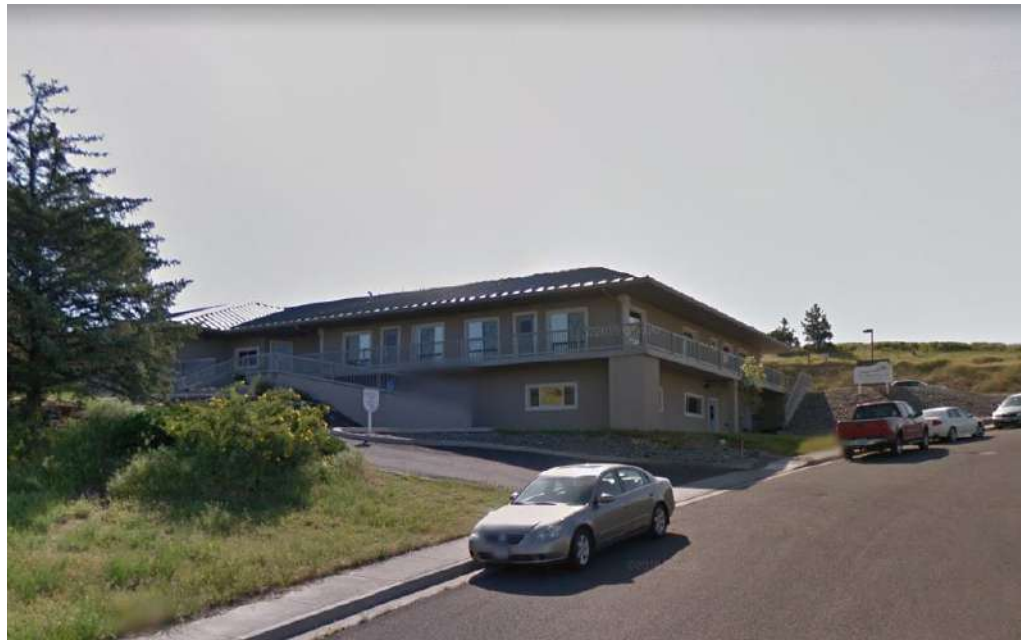
③ VIEW LOOKING SOUTHEAST
