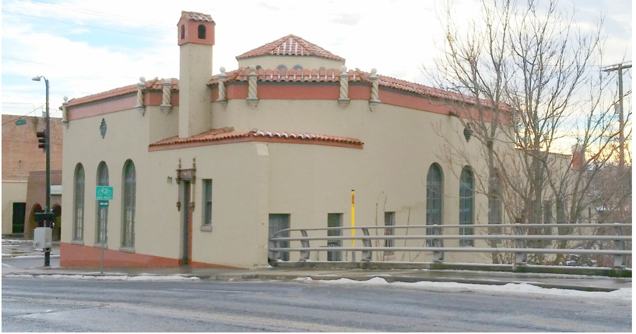
Northeast view of building at south end of Main Street bridge over Umatilla River
